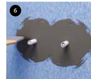
6 Cut holes for pipes, etc. Apply SCHÖNOX iFIX around the pipes.
