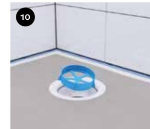
10 Position the cutting template on the JAFO floor gully. Or follow the instructions from the gully manufacturer.
