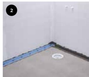
2 Cut suitable lengths of WetStop Sealing Tape. Apply SCHÖNOX iFIX and mount Sealing Tape KL. For Sealing Tape SH: mount directly on floor/wall angle. Overlap Inner/Outer Corners.
