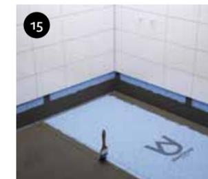
15 Glue and seal the overlaps/joints with SCHÖNOX iFIX.
