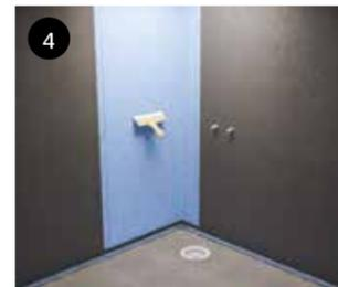
4 Use the 'WetStop Gnidde' trowel to smooth the WetStop WSF foil and press it firmly in place. Overlap the sections up to the black lines. Glue and seal all overlaps with SCHÖNOX iFIX. Where the walls meet the floor, glue and seal to a distance of 15 cm out onto the floor and up the wall.
