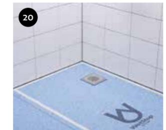
20 When all is dry (after about 3 hours), the tiles can be installed.
