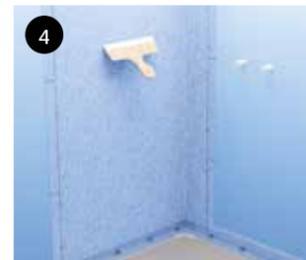
4 Rub and press the SCHÖNOX WSF to seal with the Rubbing Tool. Cut out holes for pipes, etc.
