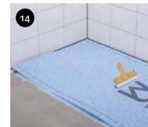
14 Rub the SCHÖNOX WSF to fix and overlap the lengths at the edges. Seal pipes in floor in the same way as for walls
