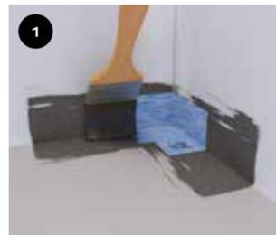
1 Clean the surface. In case of absorbent surfaces, pretreat with SCHÖNOX KH. Apply SCHÖNOX iFIX to the corner and mount Inner/Outer Corners. Press hard to fix.
