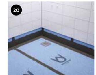
20 Once everything is dry (after approx. 3 hours), you can install the ceramic floor tiles. To finish, install the final row of tiles along the walls.
