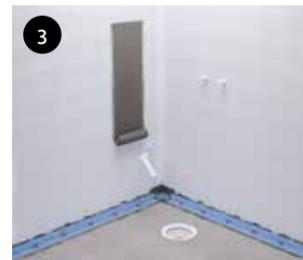
3 Cut membrane lengths so as to overlap the sealing tape at the floor/wall angle by 50 mm. Apply SCHÖNOX iFIX.
