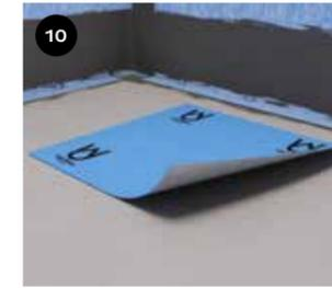
10 Remove the protective paper and mount the gully cuff. Be careful not to allow air pockets or blisters to form.
