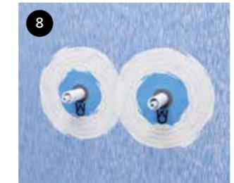
8 Mount suitably adapted Pipe Cuffs and press hard to fit. Seal the overlap by spreading surplus WetStop Foil Seal over the edge.
