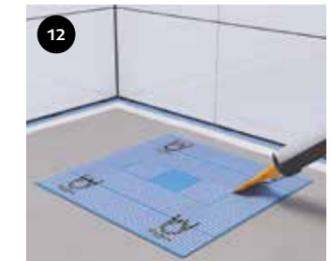
12 Cut membrane lengths so as to overlap the sealing tape. Apply WetStop Foil Seal over the cuff and Sealing Tape.
