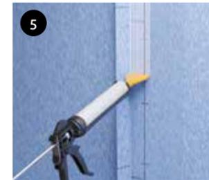
5 Overlap the lengths up to the black lines. Glue overlaps with WetStop Foil Seal.
