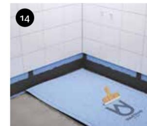
14 Rub the SCHÖNOX WSF to fix and overlap the lengths at the edges.
