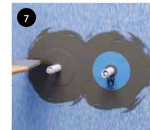
7 Mount a suitable pipe cuff and press hard to fit. Seal the edge with SCHÖNOX iFIX.
