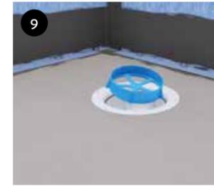
9 Position the cutting template on the JAFO floor gully. Or follow the instructions from the gully manufacturer.
