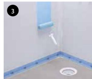
3 Cut membrane lengths so as to overlap the sealing tape at the floor/wall angle by 50 mm. Apply SCHÖNOX WSA to the wall and Foil Seal to the Sealing Tape.
