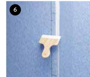
6 Seal overlaps/joints by spreading surplus WetStop Foil Seal over the edge.
