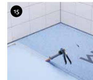
15 Glue overlaps with WetStop Foil Seal. Seal the overlap by spreading surplus WetStop Foil Seal over the edge.
