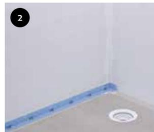
2 Apply Foil Seal and install Sealing Tape KL. In the case of an absorbent surface, SCHÖNOX WSA can be used instead. For Sealing Tape SH: install directly on floor/wall angle.
