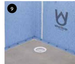
9 When all is dry (after about 3 hours), wall tiles can be installed.
