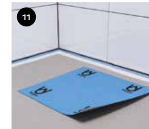
11 Remove the protective paper and mount the gully cuff. Be careful not to allow air pockets or blisters to form.
