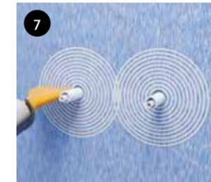
7 Apply WetStop Foil Seal round pipes.
