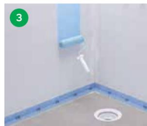
Cut membrane lengths so as to overlap the sealing tape at the floor/wall angle by 50 mm. Apply WetStop Adhesive to the wall and Foil Seal to the Sealing Tape.
