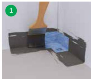
1 Clean the surface. In case of absorbent surfaces, pretreat with Casco Primer. Apply WetStop iFIX to the corner and mount Inner/Outer Corners. Press hard to fix.
