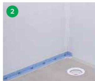
Apply Foil Seal and install Sealing Tape KL. In the case of an absorbent surface, WetStop adhesive can be used instead. For Sealing Tape SH: install directly on floor/wall angle.
