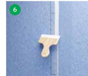
Seal overlaps/joints by spreading surplus WetStop Foil Seal over the edge.
