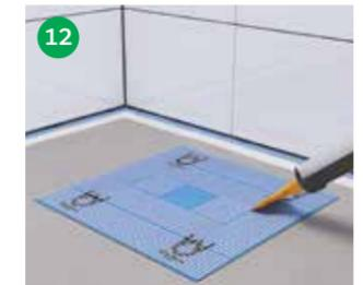
Cut membrane lengths so as to overlap the sealing tape. Apply WetStop Foil Seal over the cuff and Sealing Tape.
