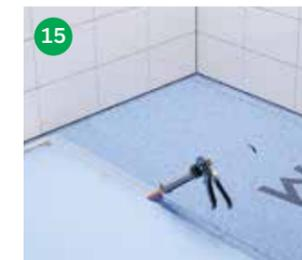
Glue overlaps with WetStop Foil Seal. Seal the overlap spreading surplus WetStop Foil Seal over the edge.
