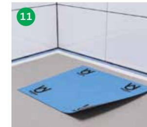
Remove the protective paper and mount the gully cuff. Be careful not to allow air pockets or blisters to form.
