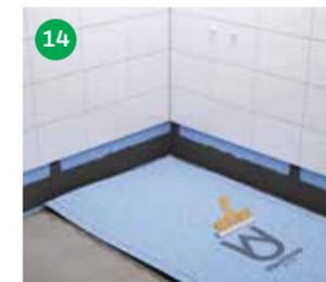
14 Rub the WetStop Foil to fix and overlap the lengths at the edges.
