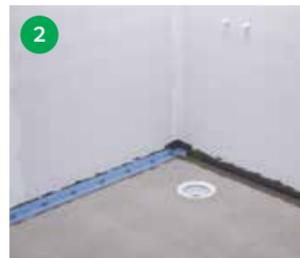
2 Cut suitable lengths of WetStop Sealing Tape. Apply WetStop iFIX and mount Sealing Tape KL. For Sealing Tape SH: mount directly on floor/wall angle. Overlap Inner/Outer Corners.
