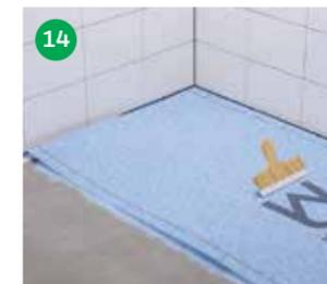
Rub the WetStop Foil to fix and overlap the lengths at the edges. Seal pipes in floor in the same way as for walls
