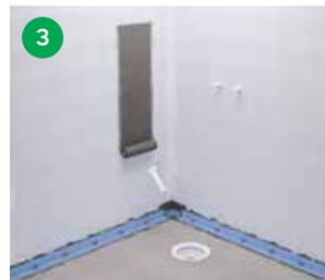
3 Cut membrane lengths so as to overlap the sealing tape at the floor/wall angle by 50 mm. Apply WetStop iFIX.
