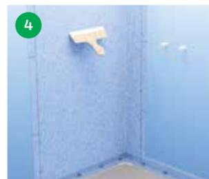
Rub and press the WetStop foil into position with the Rubbing Tool. Cut out holes for pipes, etc.
