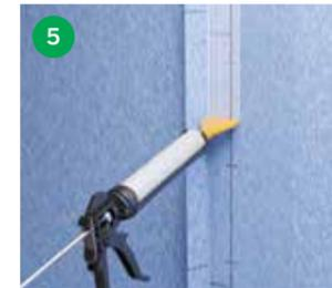
Overlap the lengths up to the black lines. Glue overlaps with WetStop Foil Seal.
