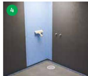
4 Use the 'WetStop Gnidde' trowel to smooth the WetStop foil and press it firmly in place. Overlap the sections up to the black lines. Glue and seal all overlaps with WetStop iFIX. Where the walls meet the floor, glue and seal to a distance of 15 cm out onto the floor and up the wall.
