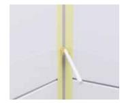
Apply sealant to the corners and the floor/wall angle to create a flexible joint. Use Sanitary Silicon or AquaSeal, while masking tape will ensure your edges are straight. Smooth the sealant with a dampened smoothing tool or finger. For dampening, use water with a drop of washing-up liquid/soap.
