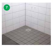
When all tiles are in place, the adhesive must be allowed to dry thoroughly before grouting.
