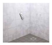
Clean off the grout with a damp sponge before it starts to dry (approx. 10-30 min.) Clean the tiles with a damp sponge. Clean diagonally to avoid hollowing out the joints. Remember to allow the grout to become finger-dry before cleaning the tiles for the first time.
