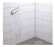
Apply the grout diagonally across the tiles with a grouting float/squeegee. Make sure the joints are generously filled. Mix the grout in the correct mixing ratio and make sure the colour pigment is mixed in. Allow the grout to rest for about 5 min. and then whip up again.
