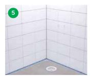
If you choose to mount a tanking membrane on both walls and floors before installing tiles, it is important to avoid holing the membrane, e.g. when laying the floor.
