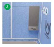
Comb out the tile adhesive. Mount the tiles before the tile adhesive on the substrate has dried, to ensure the tiles will hold properly. Avoid grouting the corners, as these need to be treated with sealant.
