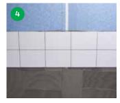
Press the tile down with a slight twist. Use tile spacers, mason line, etc., for an extra neat and even effect. Check that the rear is covered with adhesive.
