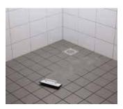
Avoid leaving grout on the tiles as it will easily become too hard to remove. Do not grout too large an area at a time.
