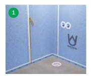
Measure the room for optimum tile cutting. Avoid small partial tiles. If possible, mount partial tiles where they will not be directly visible.
